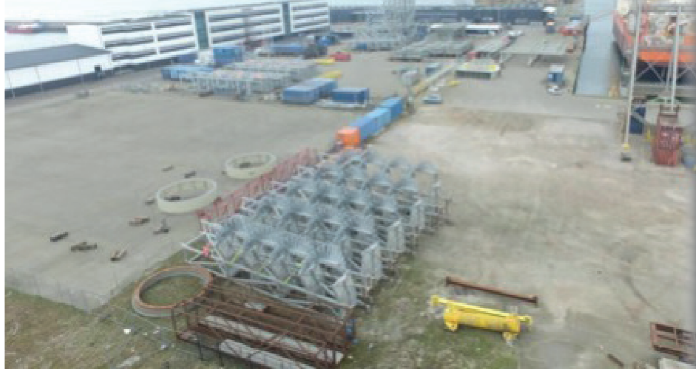
FRED OLSEN WINDCARRIER - 2018 PREFABRICATION OF 270 TON SEA FASTENING FOR THE BORKUM RIFFGRUND 02 PROJECT.
